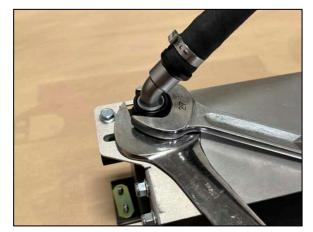
Shroud Installs: Remove the two (2) M6x1.0x25mm bolts on the top side of the shroud that were used to hold the shroud in place. Install the final two rubber isolators on the top side of the oil cooler shroud. These will get sandwiched in between the shroud and the oil cooler bracket.
